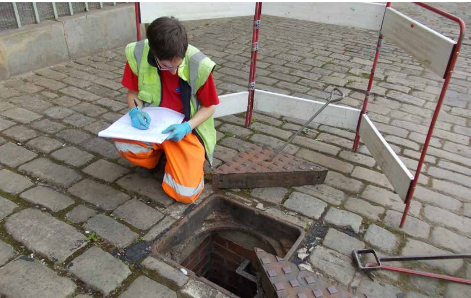
A utility surveyor carrying out a Type A survey.
