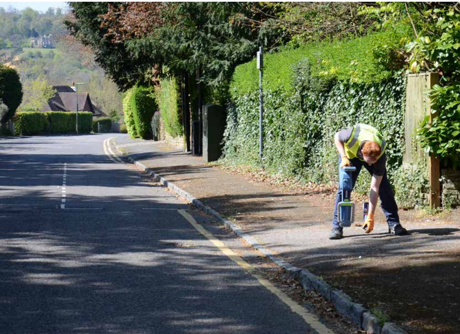
A utility surveyor using an electromagnetic locator.
